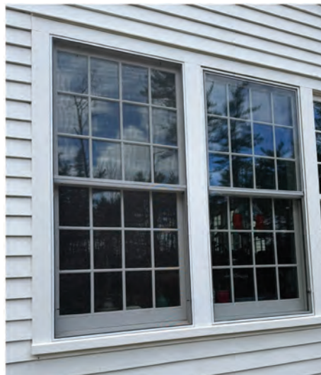
On the left, a single glass window with standard screen and a U-value of 0.86 (R=1.16). On the right, a single glass window with ThermalScreen with a U-value of 0.34 and R=2.94.
